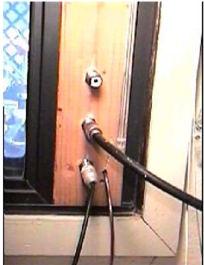
The right way to do it. Air tight and mouse tight.
